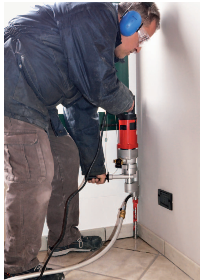
FLUSH TO THE WALL DRILLING
