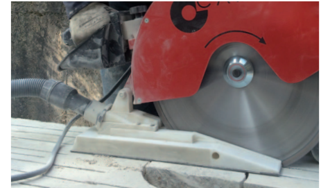
Dry cutting in reinforced concrete
