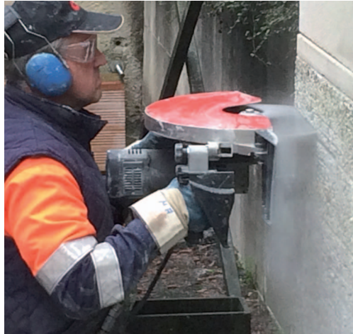
Wet cutting in reinforced concrete
