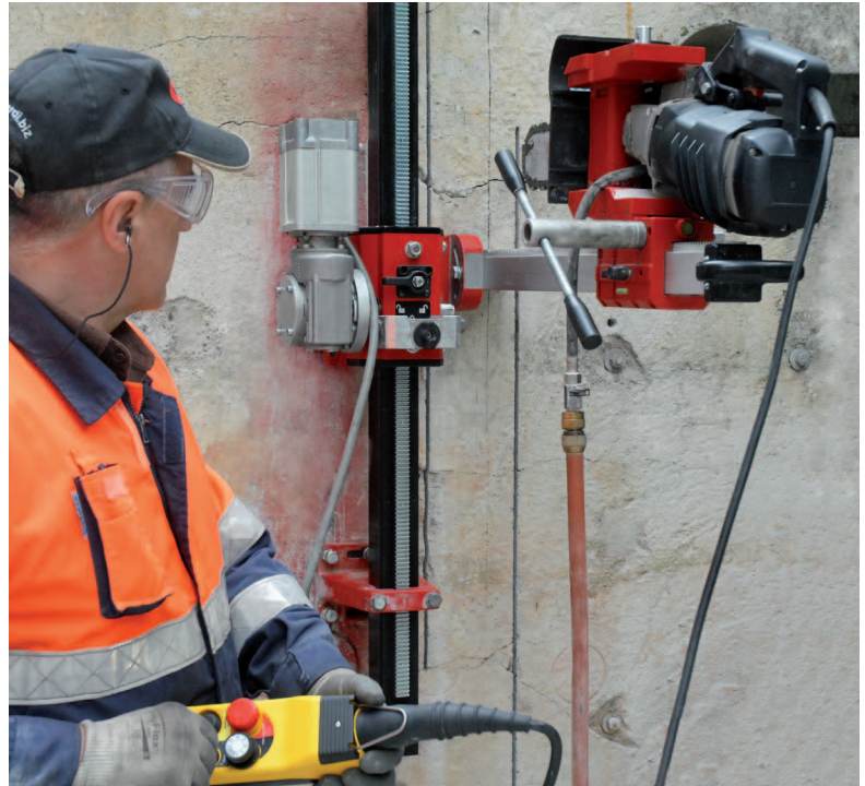
Cutting with the DV CD35-1500 using the semi-automatic feeding system DA VINCI SERVO (see pag. 21)
