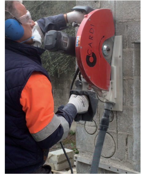
Dry cutting in concrete blocks wall
