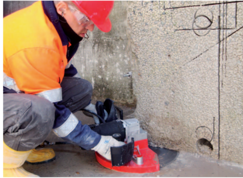
Flush floor cutting
