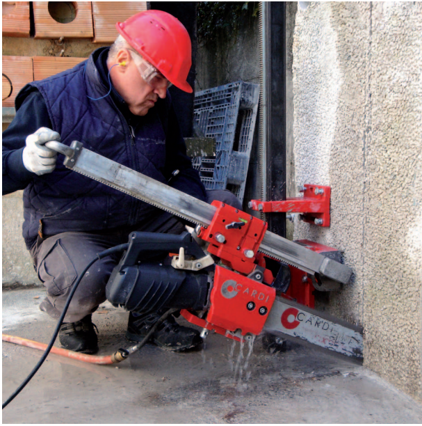
Finishing of a vertical cut till going flush to the floor, in a reinforced concrete wall.
