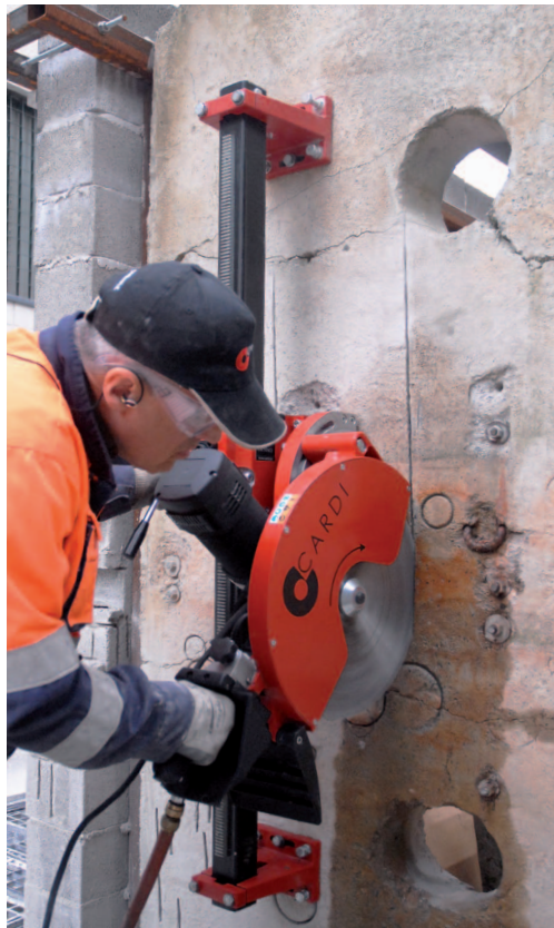
Making a vertical opening on a concrete wall
